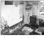
that caused the fire. At right, the burn pattern on the wall shows where the fire began behind a bed.
