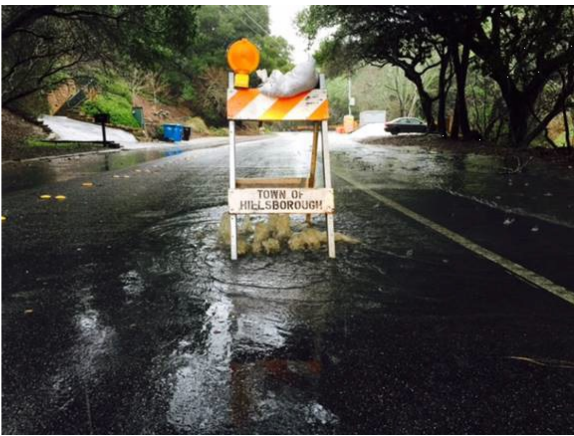
Sewer overflow before the project.
