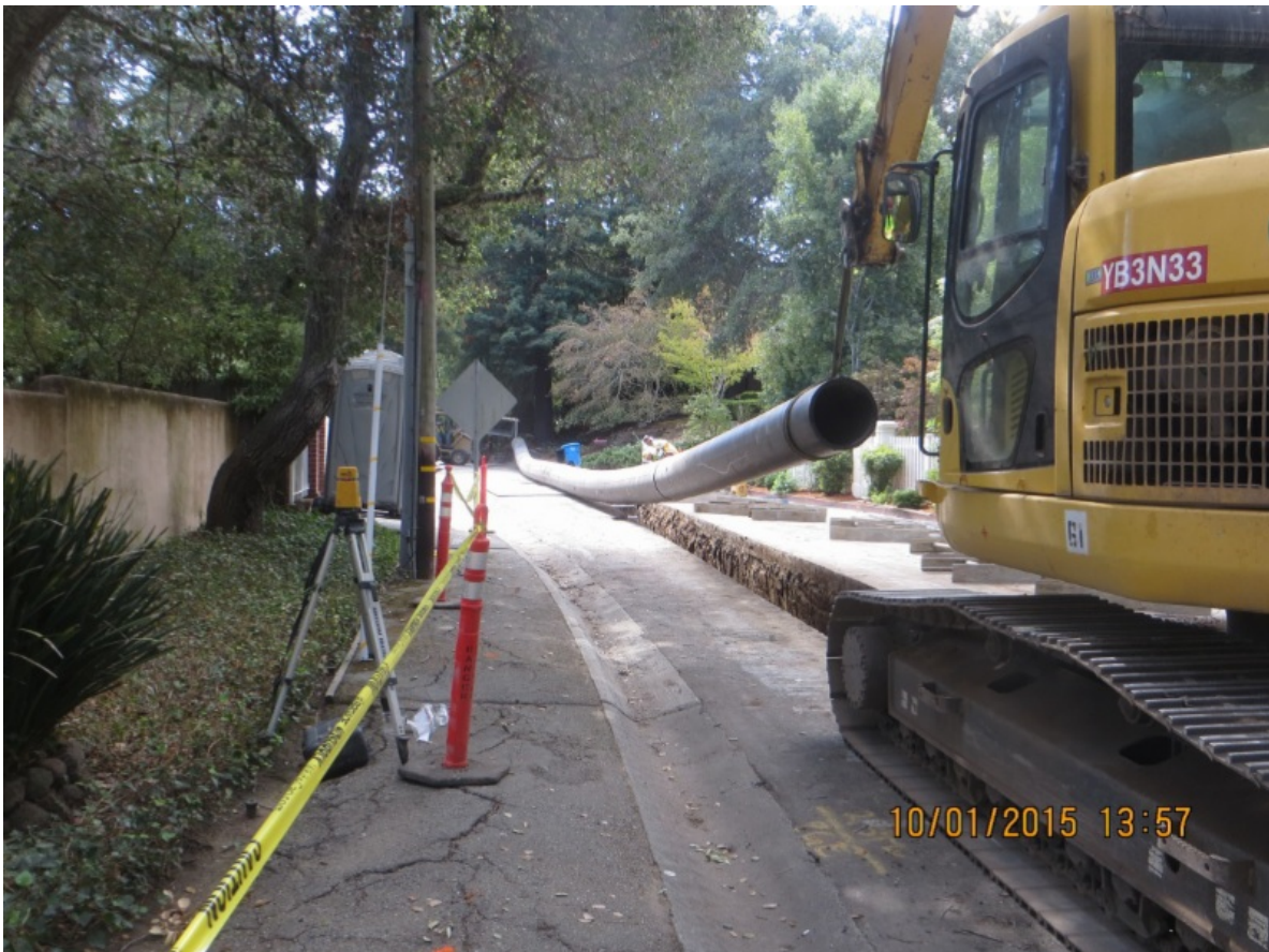
New sewer pipe being installed.
