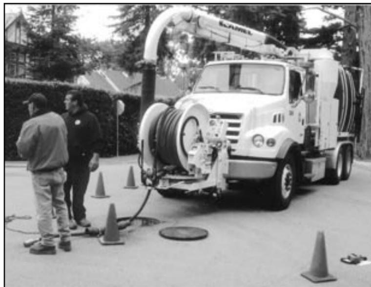
gallons of water that is shot out through the nozzle at 2,500psi (pounds per square inch) to move the nozzle through the pipe, clearing it, until it reaches the next manhole cover approximately 300 feet away. Another crewman stands at the second location and listens for the approaching nozzle. As it reaches the opening, he alerts via radio the truck crew who stop the water and reel in the hose. All clear. Future problems averted.
