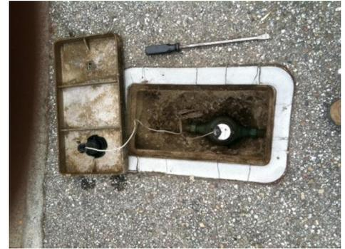
**Watch the meter.** Your meter will have a black triangular, or a red round disc that is commonly called a “leak indicator.” (Below are images of the 3 types of meters currently in use depending on the size of your water service.)
