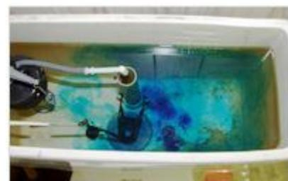
Wait 15-30 minutes. If the water in the bowl changes colors, the flapper valve needs to be replaced
