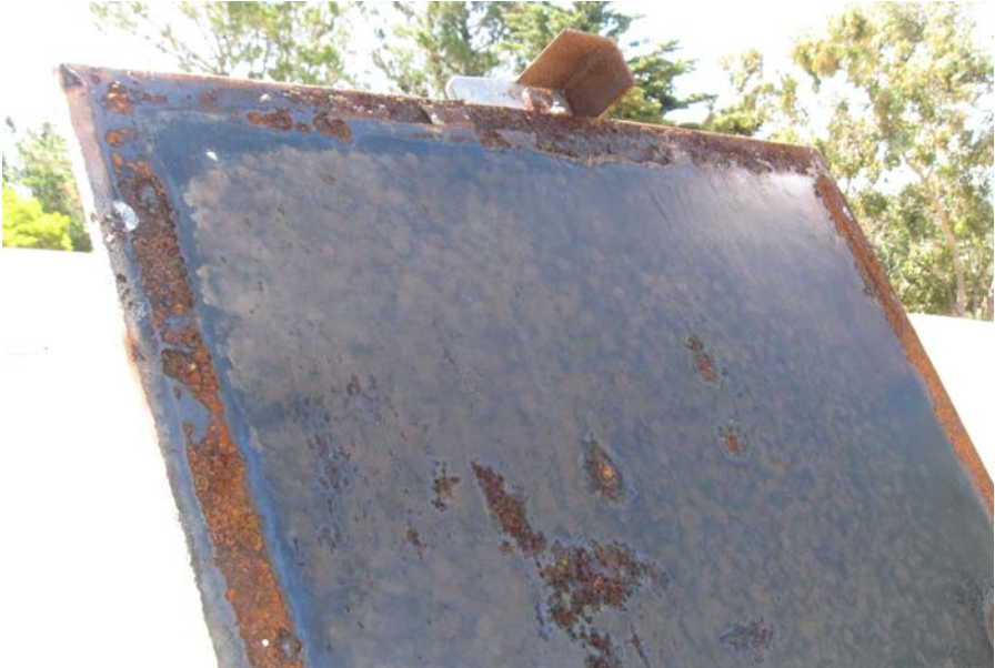
Figure 2: Underside of Roof Hatch
